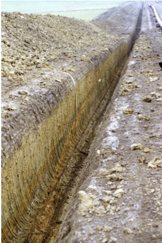
Slip plane features evident in trench below SW53: view downslope (left) profile view (centre), view upslope (right)
